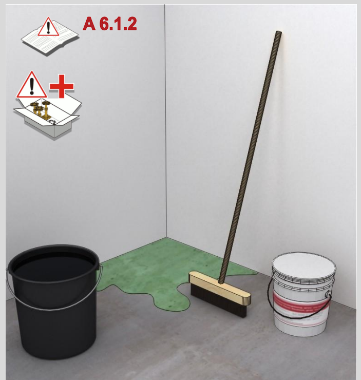
Figure 5 Application of the subfloor sealing
