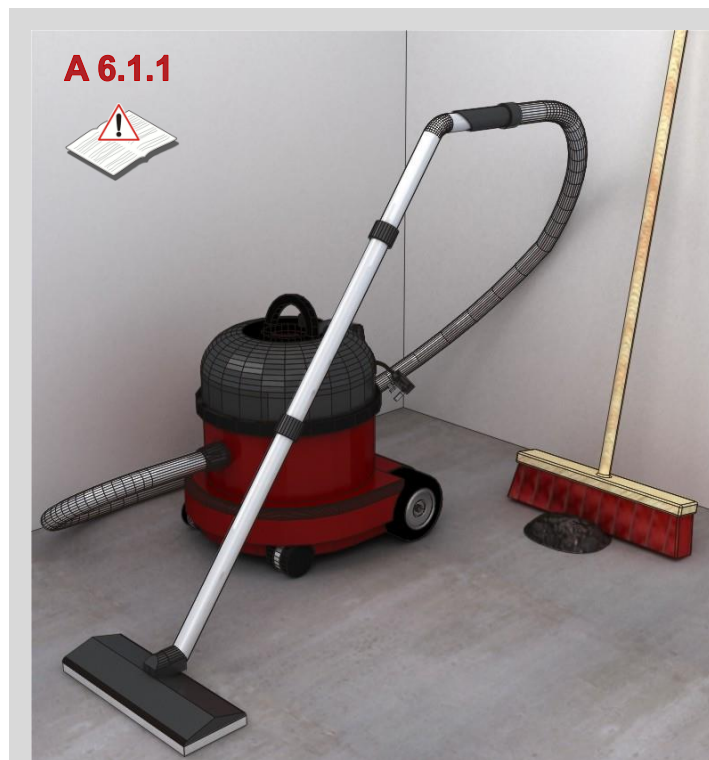
Figure 4 Cleaning of the subfloor
